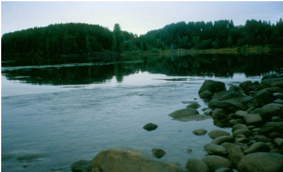
Figure 10. Confluence of the bypass channel (right) and powerhouse outflow channel (left). Water velocities and flow volume at the mouth of the bypass channel are low compared to the powerhouse outflow channel.
