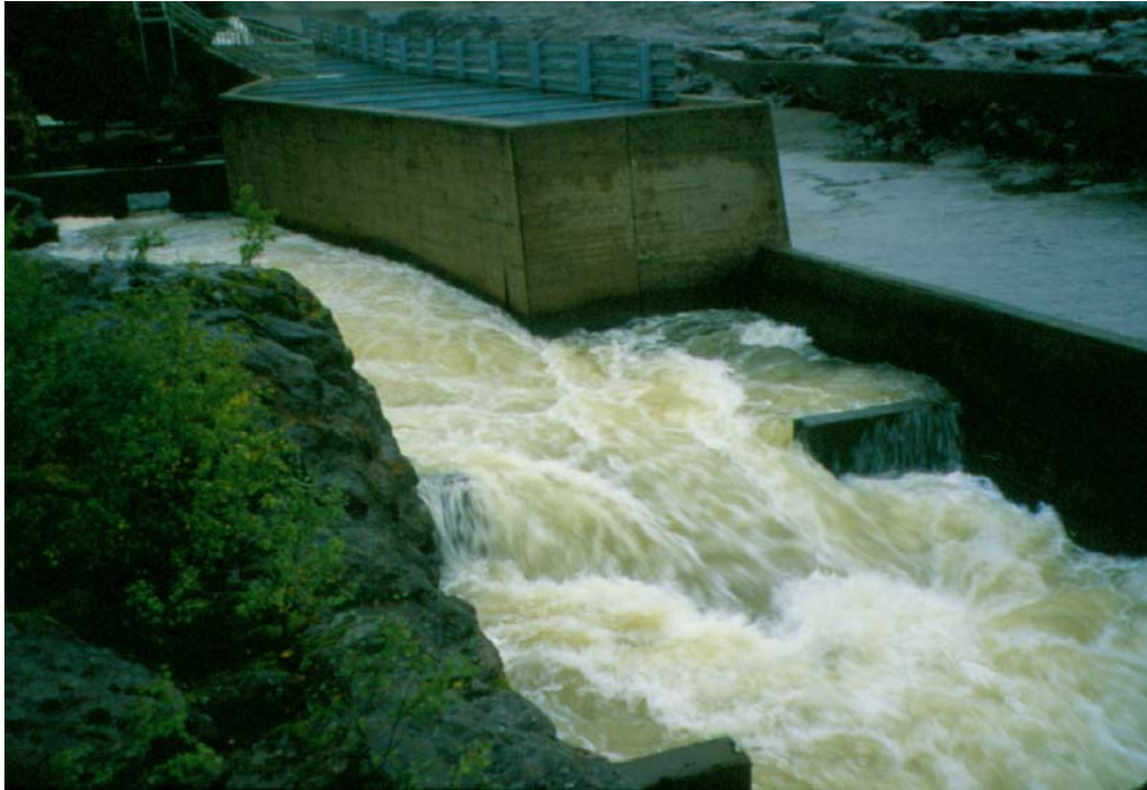
Figure 3. Norrfors Dam fish ladder entrance in upper left of photo and auxiliary water supplied to weirs downstream of the ladder entrance showing aerated, turbulent flow.
