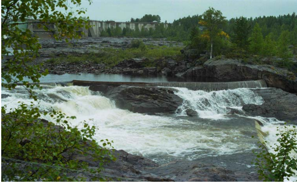
Figure 9. Laxhoppet area of natural falls and chutes has been modified to improve passage in the bypass reach under reduced flow conditions. Strategically placed weirs create 2 or 3 routes for fish passage.
