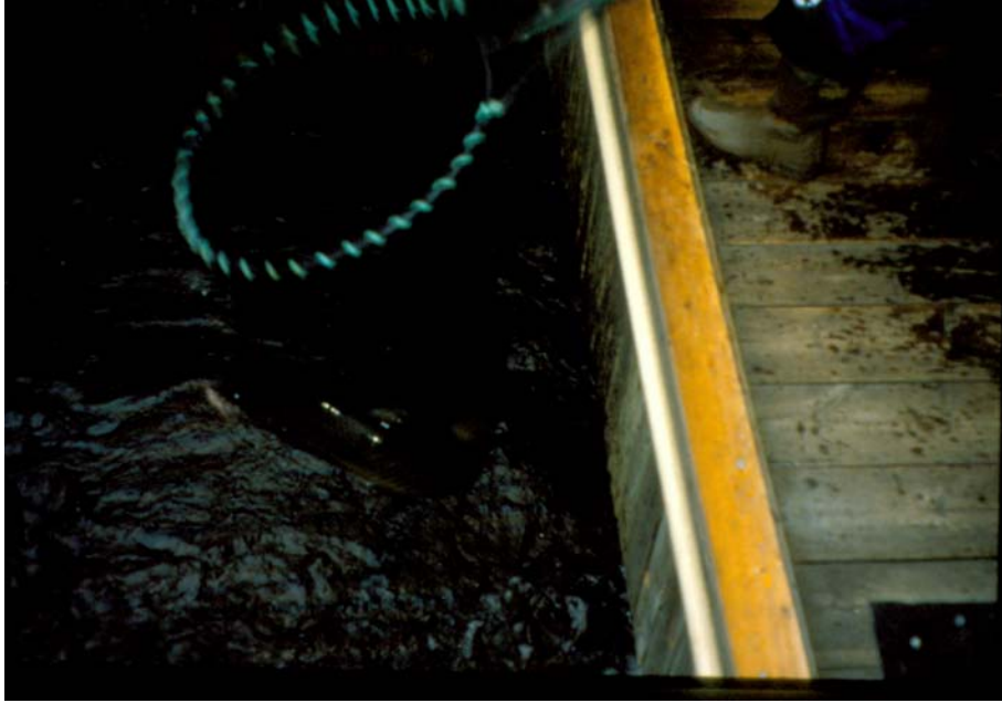
Figure 5. The adult collection facility is located in the top pool of the fish ladder. The pool is used to collect and hold fish, and the floor has a sloped brail that is raised to crowd adults for netting.
