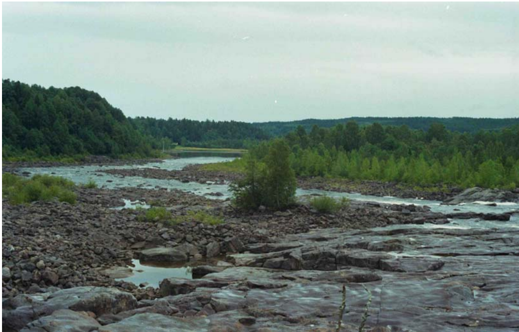
Figure 12. Lower end of the Baggböle Rapids (foreground) and bypass channel (background) under 20 \text{ m}^3/\text{s} flow. Increasing base flows through the bypass channel might improve passage conditions in the rapids and channel. The confluence of the bypass channel and powerhouse outflow channel is in the far background.
