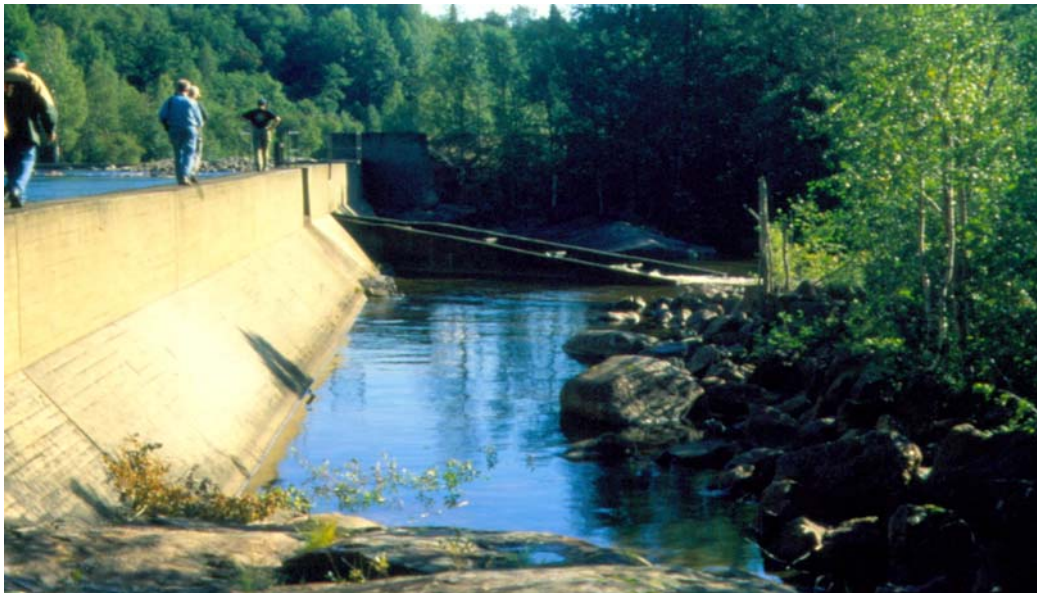
Figure 2. Small dam and ladder at the upper end of the old powerhouse headrace.
