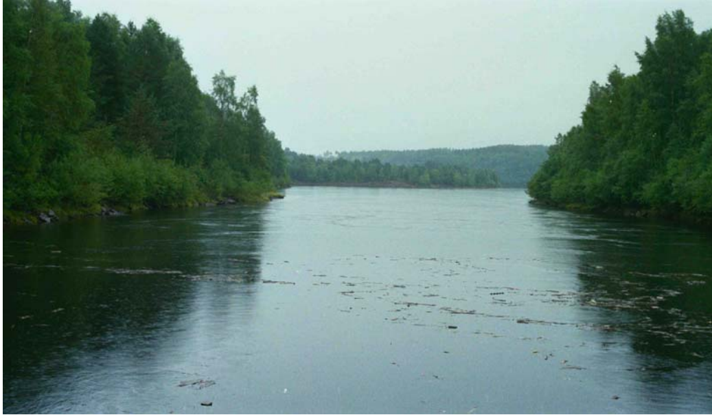
Figure 1. Stornorrfors Powerhouse tunnel tailrace, looking downstream (east).
