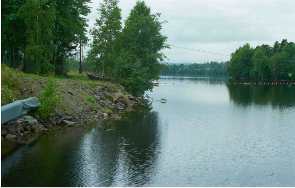
Figure 7. Fish from the adult collection facility return to the forebay via a gravity-flow, 0.3 m pipeline with flushing flow, located an estimated 75 m upstream from the Norrfors Dam. The pipe outfall is located in the area shown along the right bank of the peninsula that divides the powerhouse and spillway forebays.
