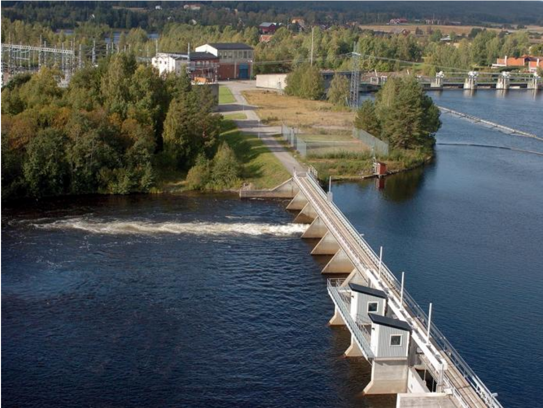
Figure 9.2 The Dönje Plant
