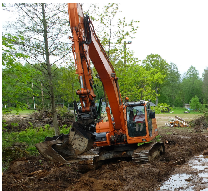
Lillån, an artificial tributary built for the Emån river at Kvillefors, Vetlanda. Initial digging for the Turefors circulation, began in June 2015.
